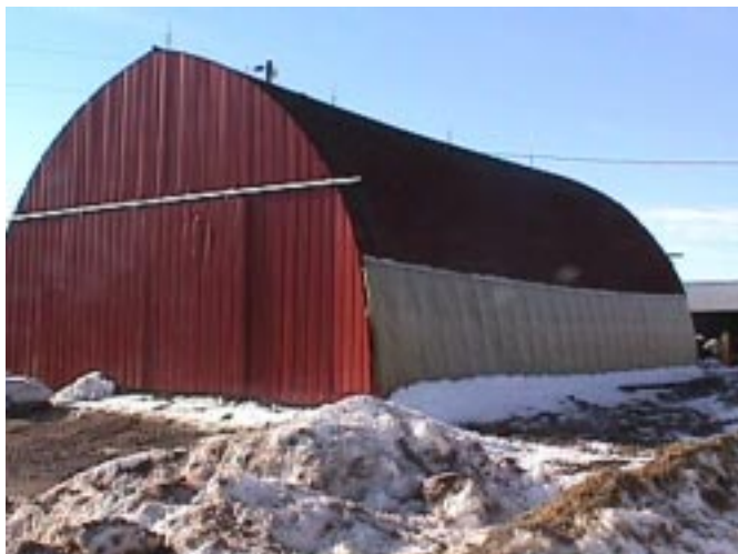
Gary Peterson, Douglas County, remodeled this Quonset type building into a curtain sided calf barn. The lower eight feet of siding of each wall was removed and a roll-up curtain was attached on the outside. Located several miles from Lake Superior, the calves have done well for two years now. The height of the building provides plenty of natural ventilation.
