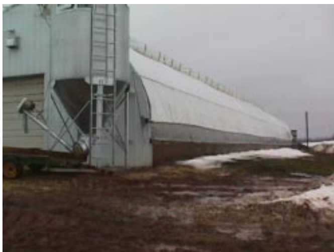
Tom Kriskovich, Ashland County, uses a greenhouse barn to raise calves and young heifers. An overshoot roof provides natural ventilation. On sunny days the calf pens are bright, and the full-length curtain is easily rolled up to maintain an even temperature. Winter snows have not been a problem for the roof.
